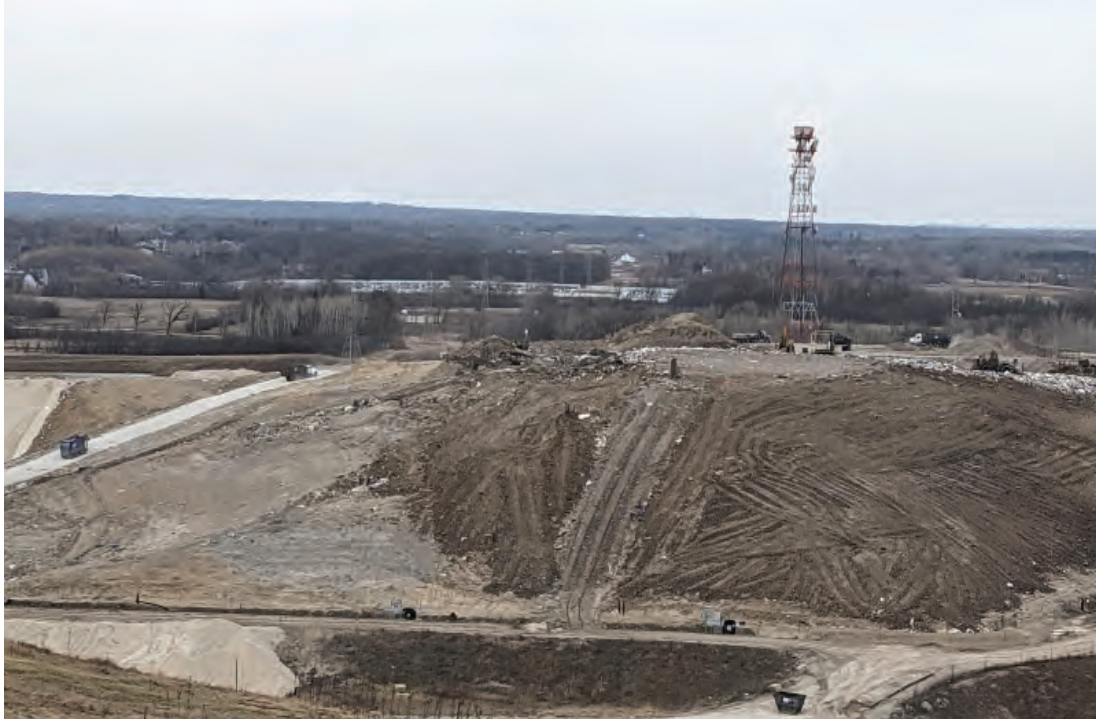
South slope of North Expansion West, fully coveredf in intermediate cover
