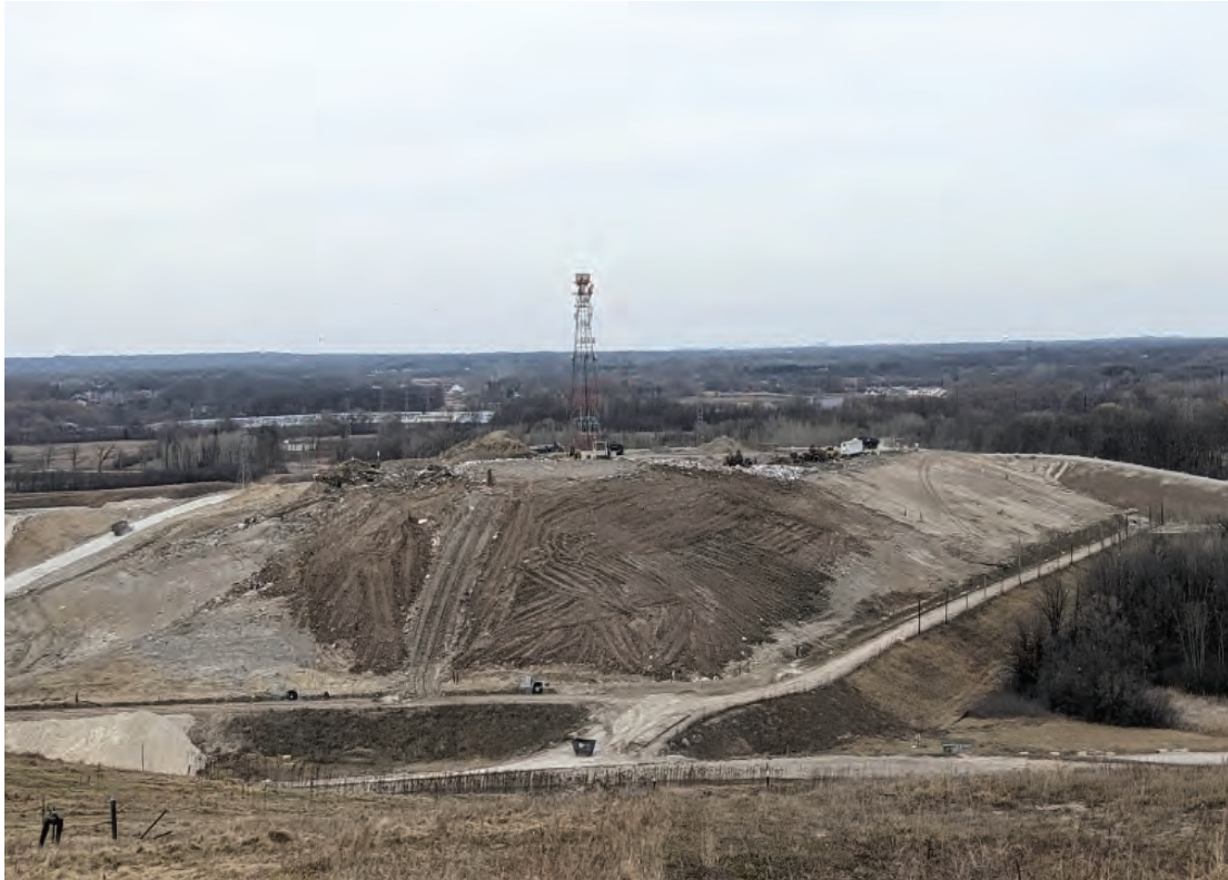
Overview of Phases 1 & 2 of North Expansion West
