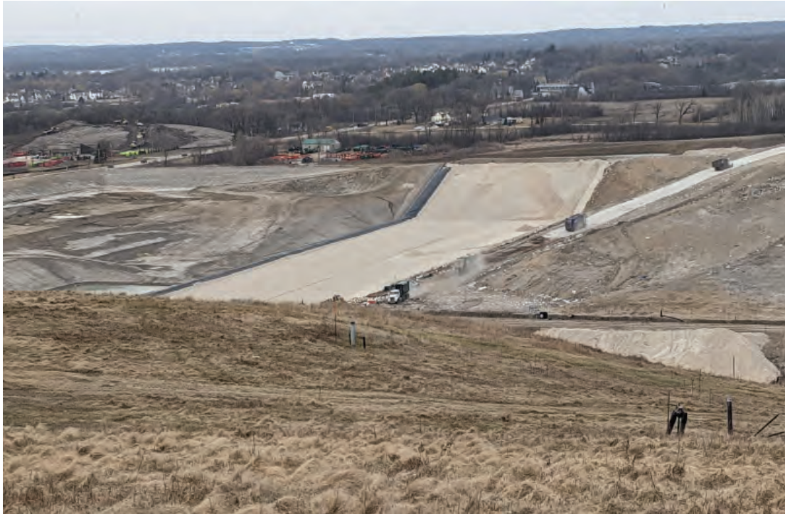
Phase 3 receiving waste, starting today. Select waste fluff layer being placed in Southeast corner
