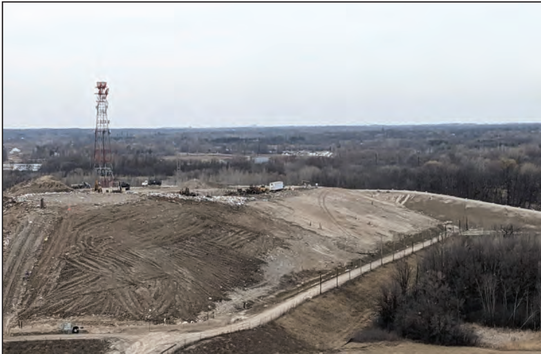
East slope of North Expansion West, fully coveredf in intermediate cover
